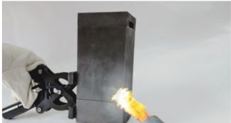
Preheat mold and conductor
